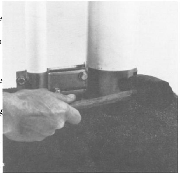
*Use a Rubber Hammer to "Shape" the Casing Adapter to the arc of the well casing.*
